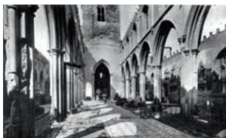
Censorship rules did not permit the British press to show bombed buildings. These three views of the bombing at London Wall, Moorgate Station and St Giles Church Cripplegate were part of a set of postcards passed by the censor in 1944.
