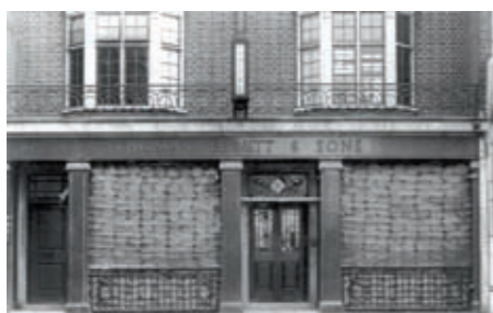
Sandbags protect the premises of Thomas Ebbutt funeral directors in Croydon
